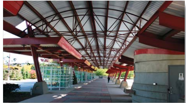
Pace will be completing a mid-life renovation to its Northwest Transportation Center in Schaumburg in 2013.
