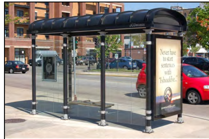
Covered bus shelters provide protection for riders
