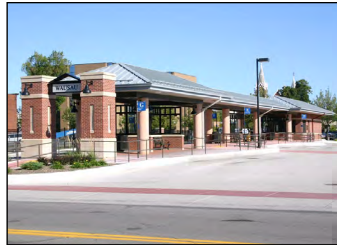
Well designed transit hub with appropriate pedestrian amenities
