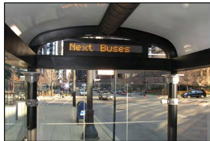
Bus shelter displaying real-time arrival/departure information
