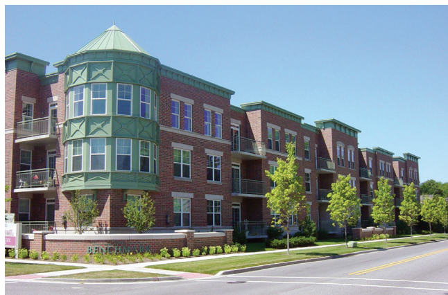
Low-rise multi-family residential building
