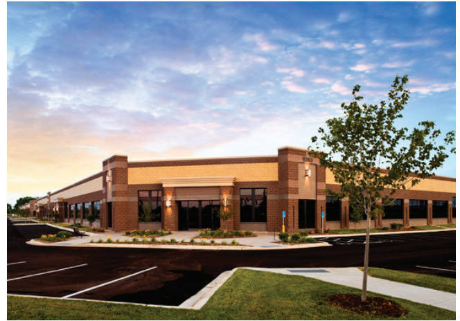
Front office entrance of a manufacturing building
