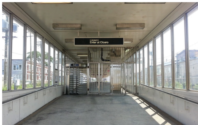
Sign directing transit customers to Cicero Avenue entrance. Source: T.Y. Lin International
