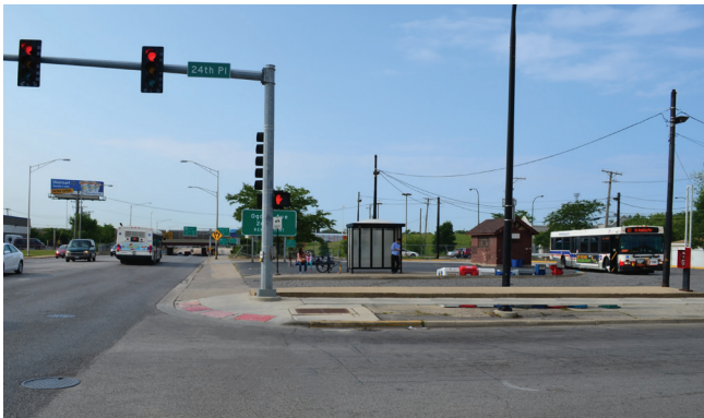
Above: Existing conditions at Cicero Avenue & 24th Place
