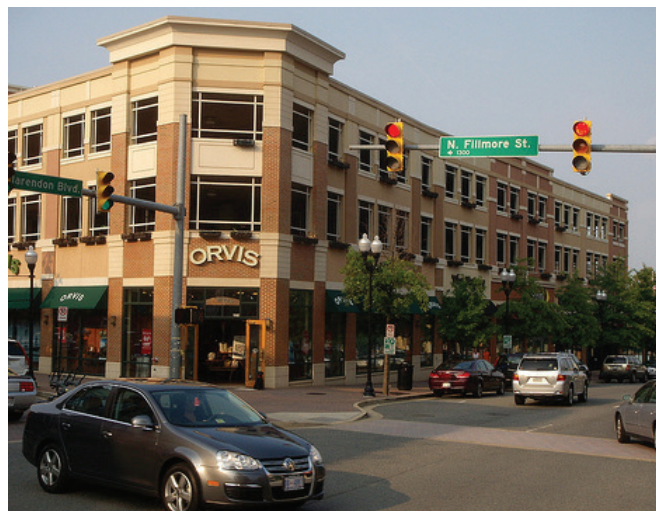
Parking structure with ground floor commercial use
