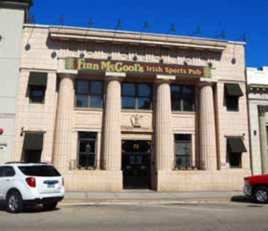
United States Bank Building / Built in 1911 (Facade: 1927) / 72 N. Williams
