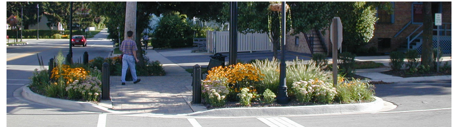
Corner 'bumpouts' improve pedestrian safety and allow for additional landscaping
