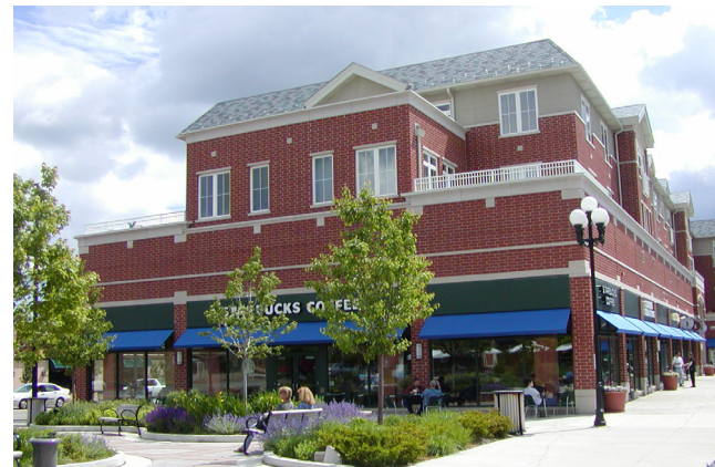
Upper-story building ‘stepbacks’ can help reduce the overall mass and scale of a building.
