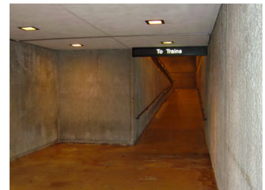
Station house interior
