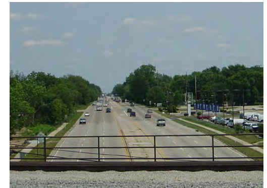
211th Street Metra Station platform (looking east)
