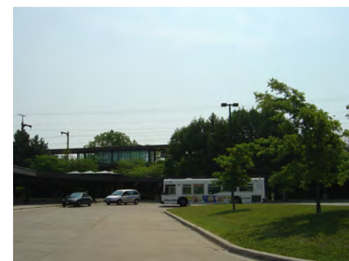
211th Street Station bus turnaround, Matteson
