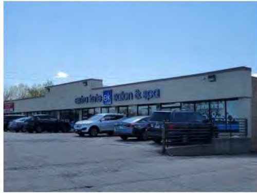
Strip Mall at 3911 Sauk Trail
