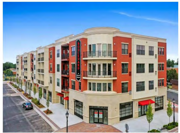
The Boulevard at Central Station (Tinley Park)
