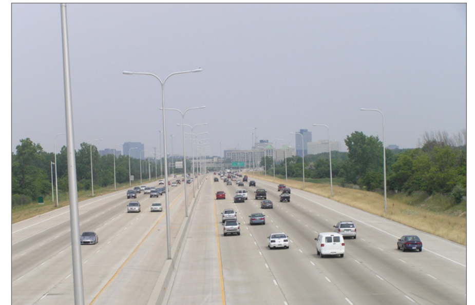
Interstate 290 at Mile Marker 4, Looking North Toward Schaumburg
