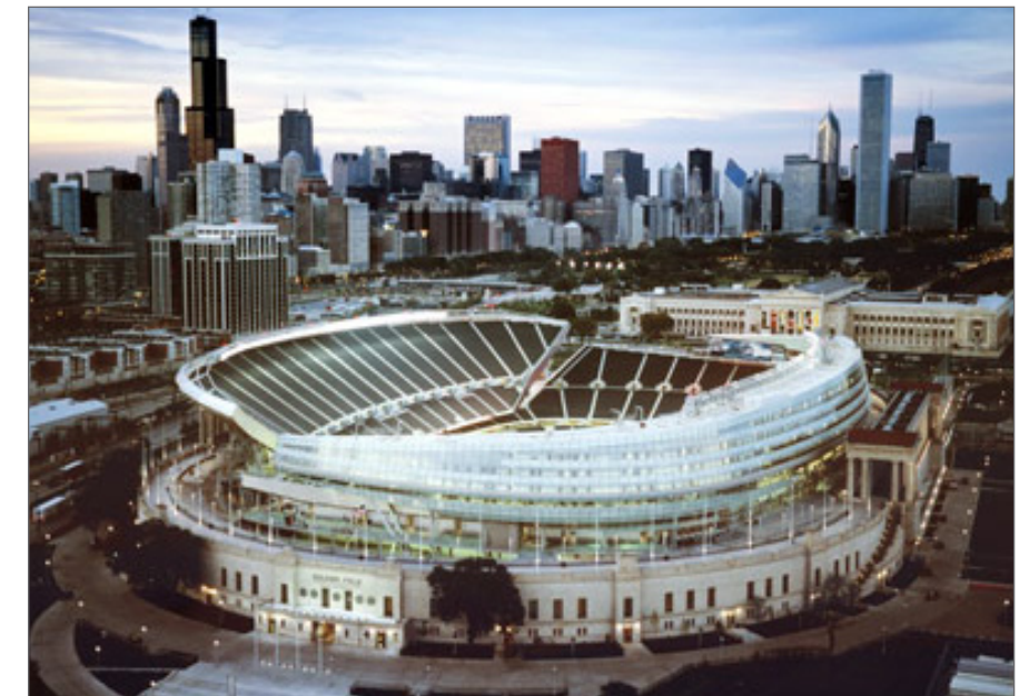
Pace Route 237 is an Express Special Events Route to Soldier Field in Chicago
