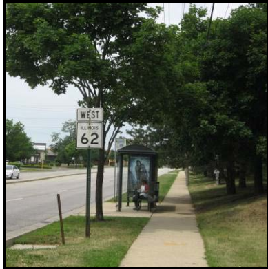
Photo 1- Good example of sidewalk leading to concrete pad
