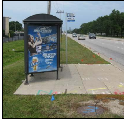
Photo 2- Example of a concrete pad with no sidewalk access
