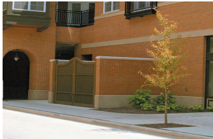
Masonry walls and decorative fencing used for service and trash receptacle screening.
