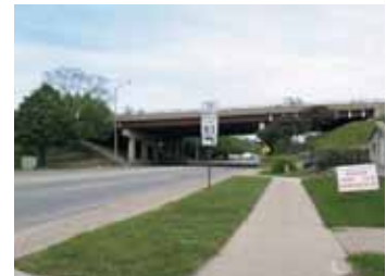
Irving Park Road underpass at Route 83
