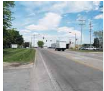
Typical County Line Road existing conditions
