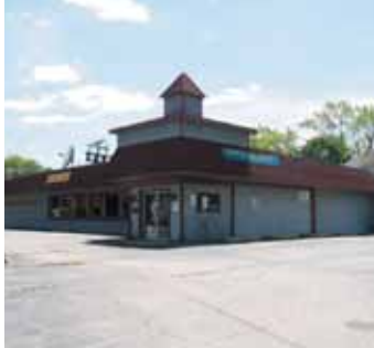
Vacant retail building on Green
