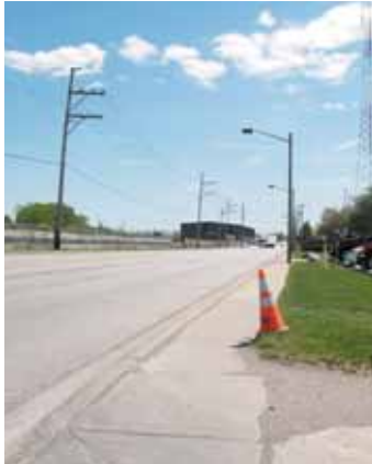
Sidewalk conditions on Green
