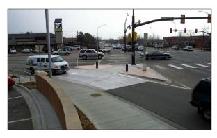
Figure 1.14: Photo showing raised channelize right-turn lane with pedestrian refuge
