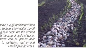
A rain garden is a vegetated depression that helps reduce stormwater runoff by filtrating rain back into the ground to maintain the natural cycle of water. A rain garden can be placed near buildings, in parkways, and in and
