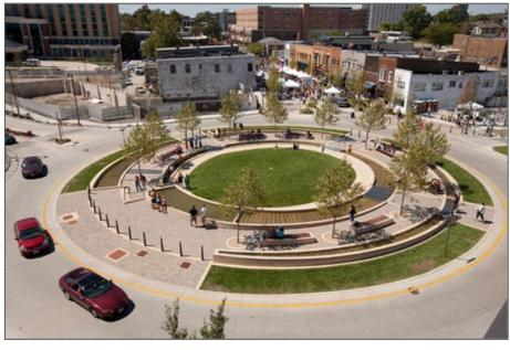
Figure 1.4: Uptown Circle, Normal, Illinois. Located in the heart of the Central Business District, the roundabout addressed community traffic issues and created an attractive public gathering place. The design is a showcase of green infrastructure with an extensive rainwater collection system below.
