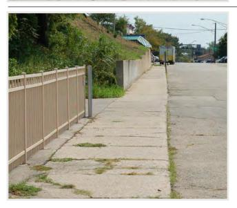
Further to the south along Nippersink Boulevard. there is a sidewalk that is in a deteriorated condition as shown. There is also a retaining wall on the east side of the roadway due to a severe slope up to the elevated commuter parking lot at the Village water tower site.
