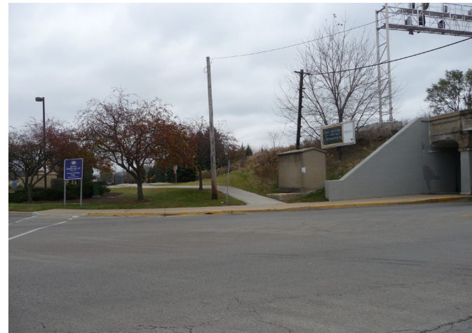
Spring Street underpass and pedestrian access to the Middle Parking Area and Metra platforms
