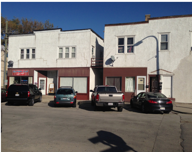
Several buildings in Site C
