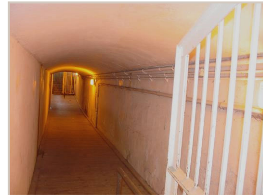
Figure 5-11, Existing Pedestrian Underpass
