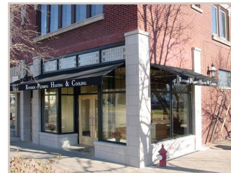
Figure 5-22, Good Example of Façade Renovation
