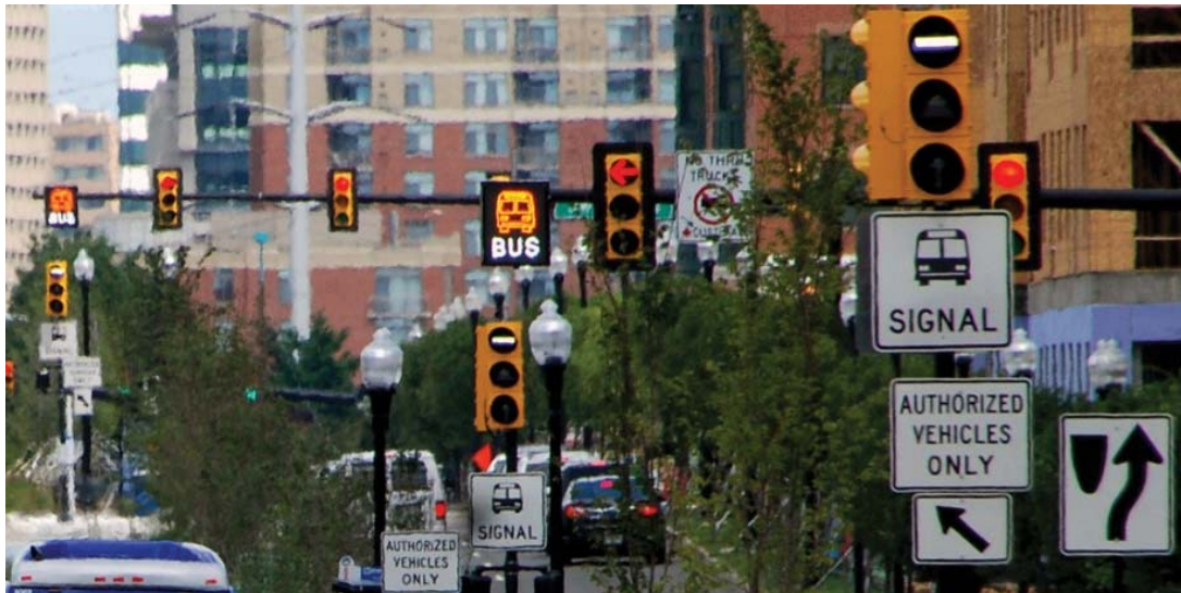
Figure 23: Example of Bus Priority Signal and Signage
