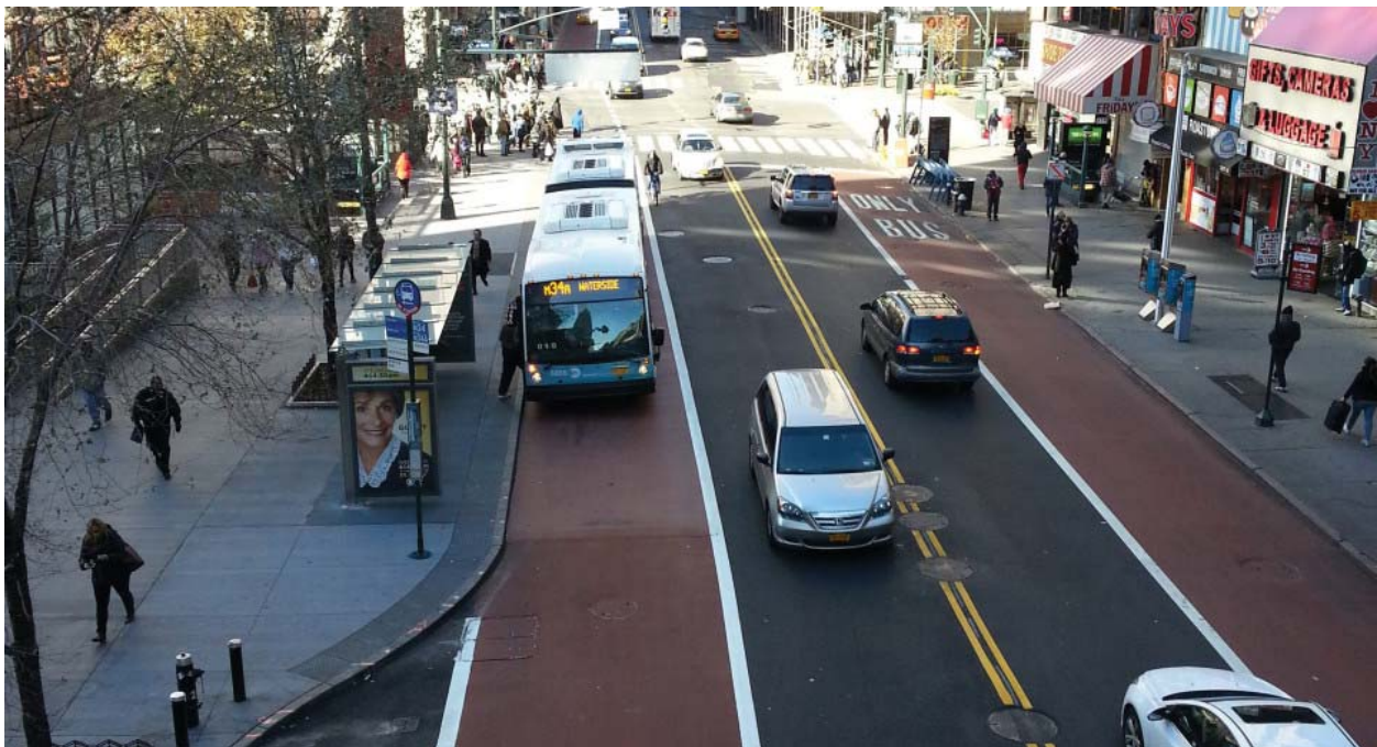
Figure 20: Example of a Dedicated Bus Lanes
