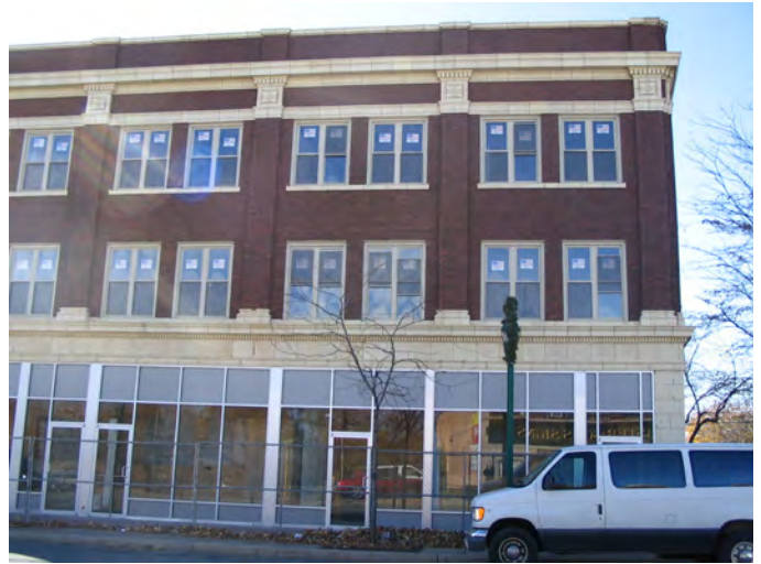
Recently renovated mixed-use building, with residential units on upper floors.
