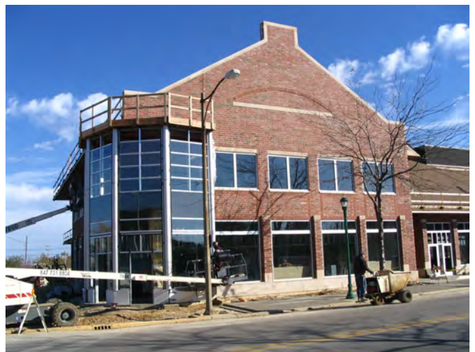
The Grant Place development, under construction as of late 2006.
