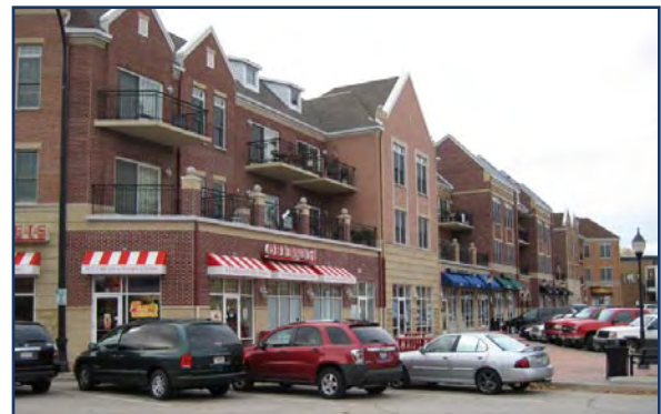
❖ A variety of roofline features are utilized on this mixed-use building, including side and front facing gables and dormers. The intermittent height setbacks of the second and third floors help further define a unique roofline.
