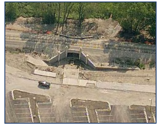
❖ Pedestrian Underpass Example, Orland Park, IL
