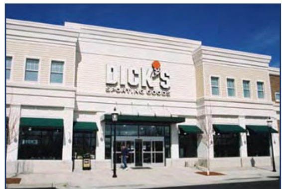
❖ Building is oriented along the public street; the prominent main entrance, decorative awnings and cornice lines provide a pedestrian-shopping atmosphere.
