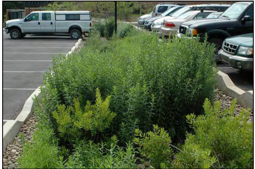
❖ Bioswale within a parking lot.
