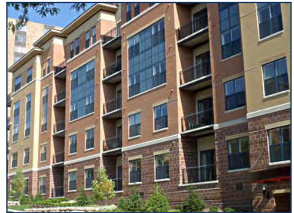
❖ Facade is composed of a mix of masonry materials, colors and textures that compliment each other. Recessed balconies help to break up the mass of the structure.
