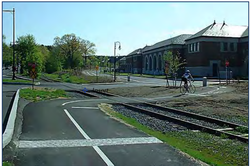
❖ Tactile warning stripes warn pedestrians and cyclists of the railroad crossing ahead.
