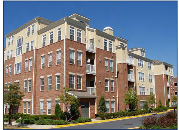
❖ Varying height setbacks work to create a dynamic roofline; also note the variety in window details, especially along the side facade.
