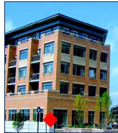
❖ Building’s front and side facades are complimentary in that the architectural features evident on the front, i.e. the horizontal banding, window divisions and height setbacks, are also apparent on the side.
