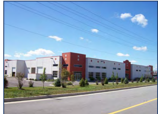
❖ Existing industrial buildings demonstrate a unified design theme; colors, materials, awnings, and window patterns are consistent.
