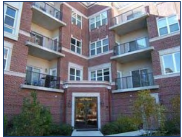
❖ Rear facade of building is defined by a consistent pattern of window fenestrations and recessed balconies.
