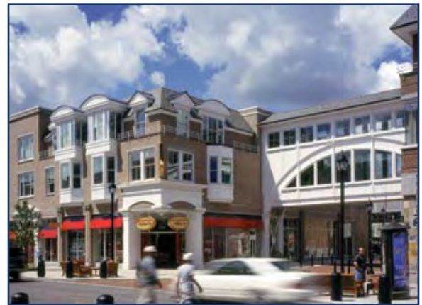
❖ The facade displays a variety of window sizes and treatments, including bay windows on the second and third stories.
