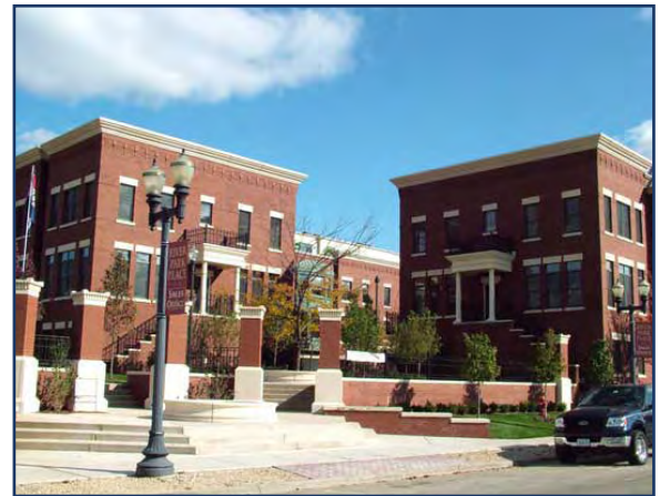
❖ Buildings maintain complimentary cornices, lintels and fenestrations; also note the colonnade architecture that is integrated into the design of the corner.
