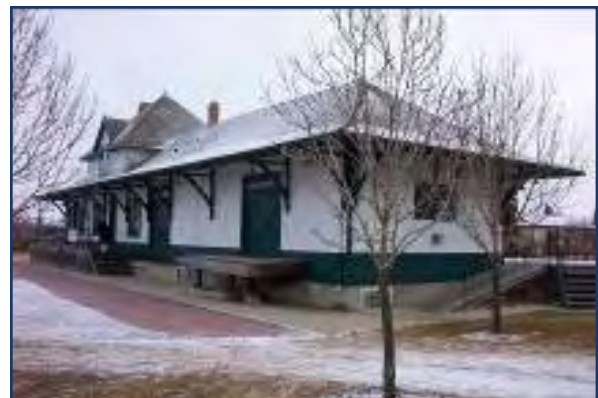
❖ Example of similar roof brackets on historic train stations in Winona, MN and Alberta, Canada.
