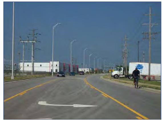
▲ 143rd Street looking west. Note lack of provision for bicyclists, and presence of existing development which will block view of proposed station.
