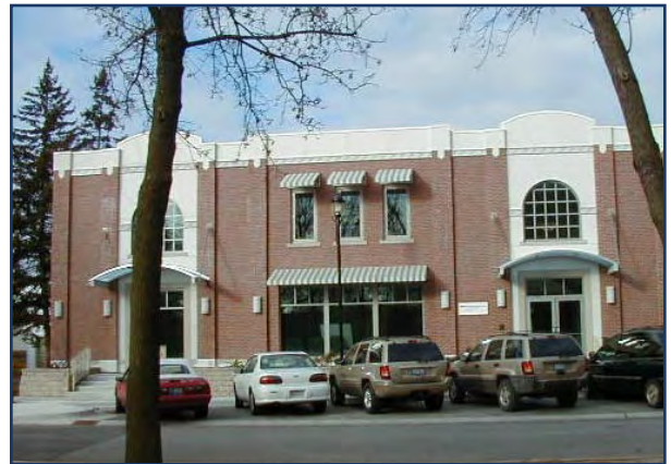
❖ Building facade demonstrates a consistent pattern of architectural detailing that includes vertical subdivisions, changes in materials and colors, as well as decorative awnings and window treatments.
