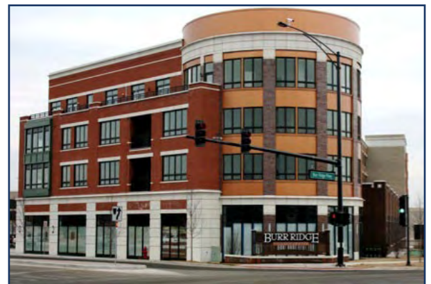
❖ A curved “edge” facade makes corner buildings distinct architecturally, while the fourth story side-setback and tiered height adds depth to the buildings mass.
