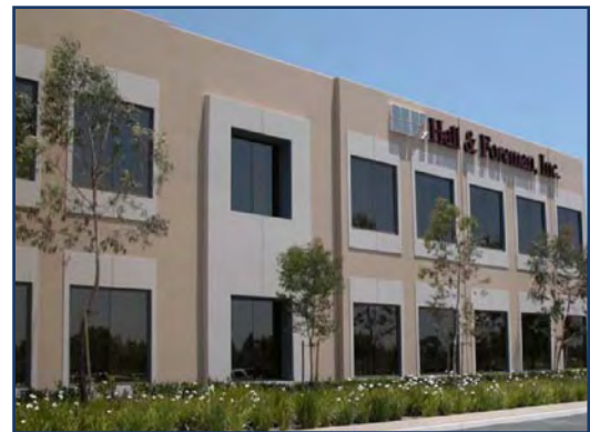
❖ Example of an industrial facade integrating complimentary colors and textures. Note: Second story windows help to divide the mass of the structure.
