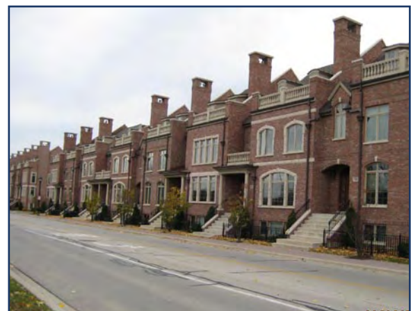
❖ Street-facing townhome façades are given definition by alternating window patterns and interspersing a variety of recessed, porch architecture. Horizontal, concrete banding helps to break-up the building mass.
