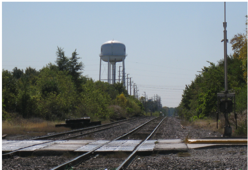
Intersection of UP/CSX railroad tracks and Sauk Trail, looking North.
