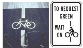
(MUCTD-approved Bicycle Detector Pavement Marking) together with a Bicycle Signal Actuation Sign can locate the appropriate place for the bicyclist to stop to actuate the signal. Quadruple loop detectors can also be installed as they are more sensitive to bicycles. Traffic signals can also be modified to provide an adequate clearance interval for bicyclists who are crossing at the end of the green.
