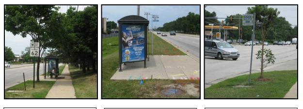
Photo 1- Good example of sidewalk leading to concrete pad
