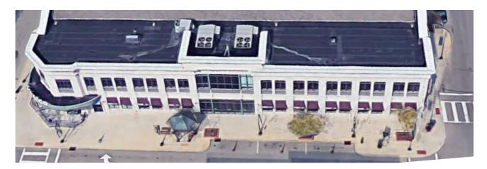
Figure 5-L. Rooftop Utilities Screened from the Street by a Parapet
