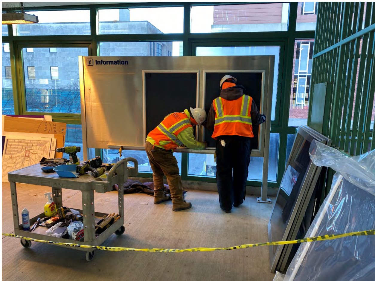
RTA maintenance contractors replacing the original stainless map frames at Davis CTA station with new aluminum snap frames.
