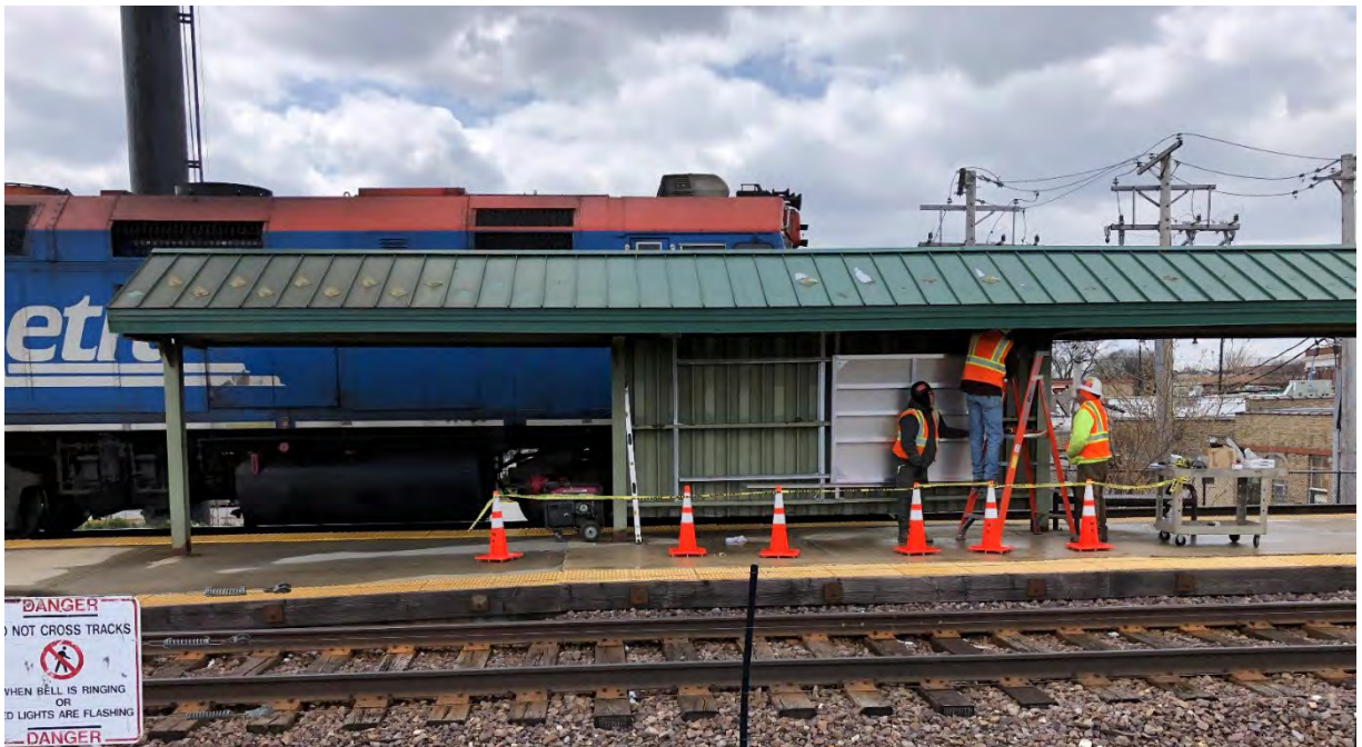
Installing the sign structure on the Metra center platform. The frame is attached to the existing wind break.
