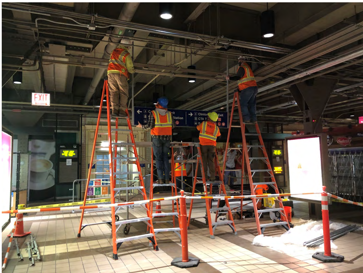
Installing a large overhead sign in the Suburban Concourse at Ogilvie Transportation Center
