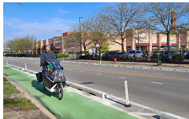
Prefabricated concrete curbs on Roscoe Avenue (CDOT)
