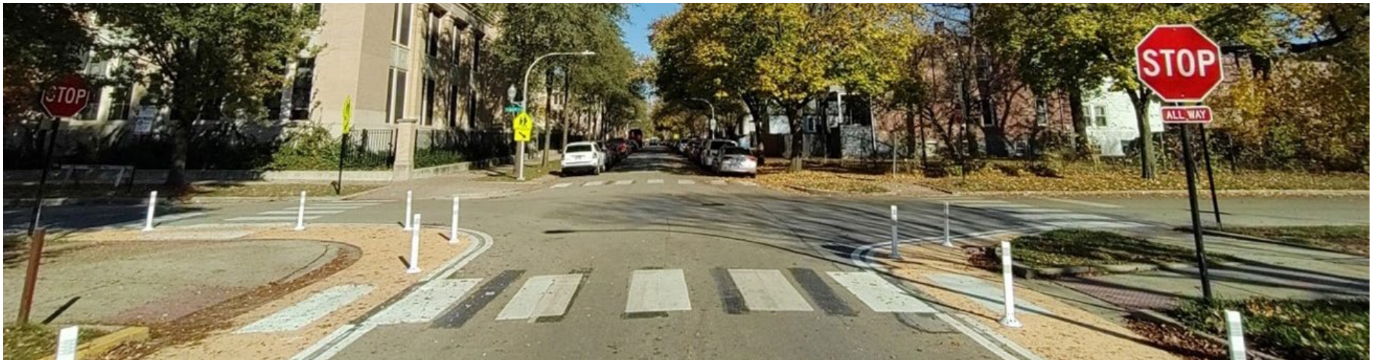
Examples of quick-build strategies include painted bumpouts and curb extensions and temporary bollards
