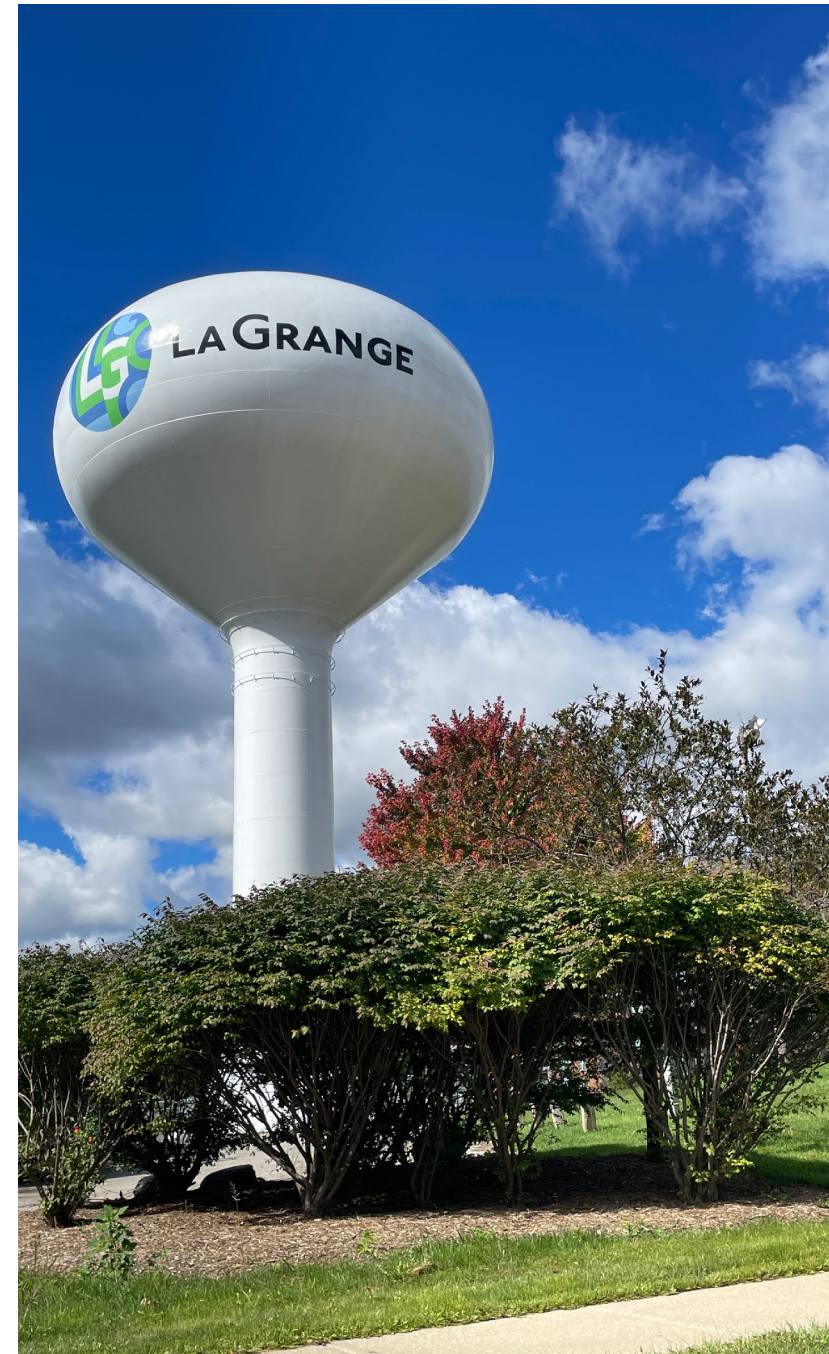
La Grange water tower
