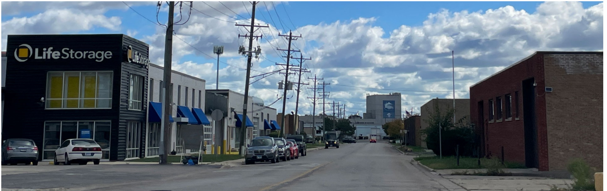
The Industrial Subareas have historically been comprised of smaller, light industrial uses
