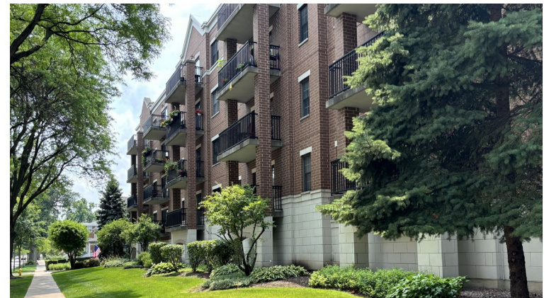
Housing in La Grange
