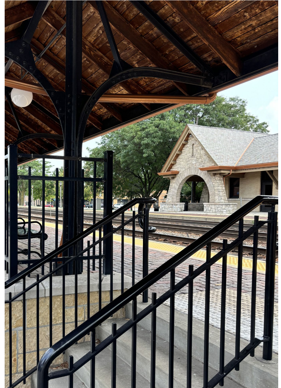
Stone Avenue Metra Station
