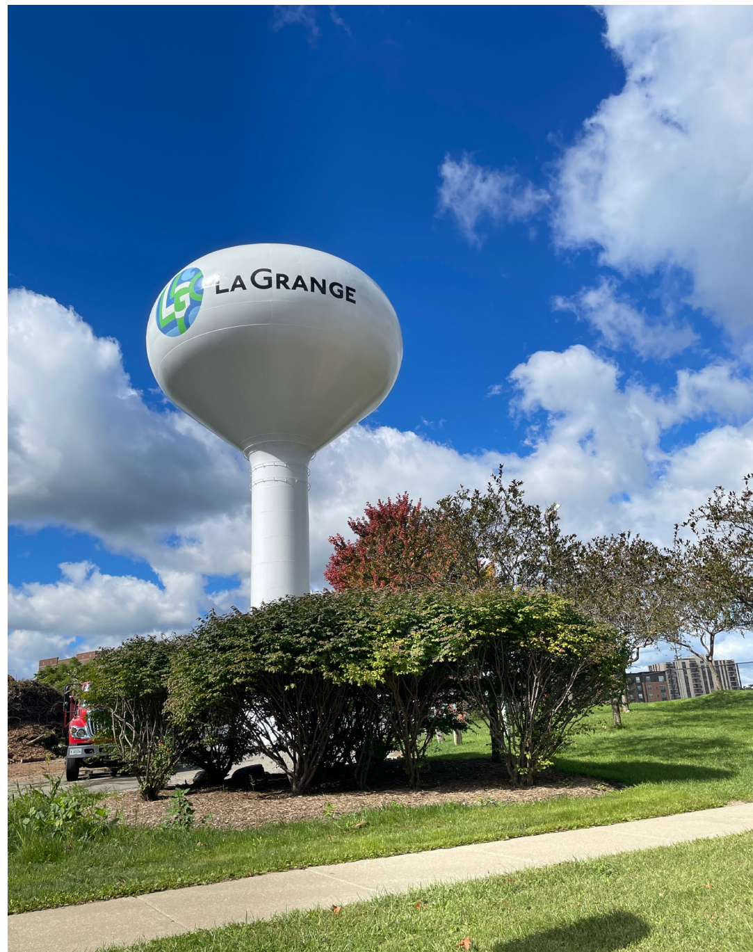
La Grange water tower
