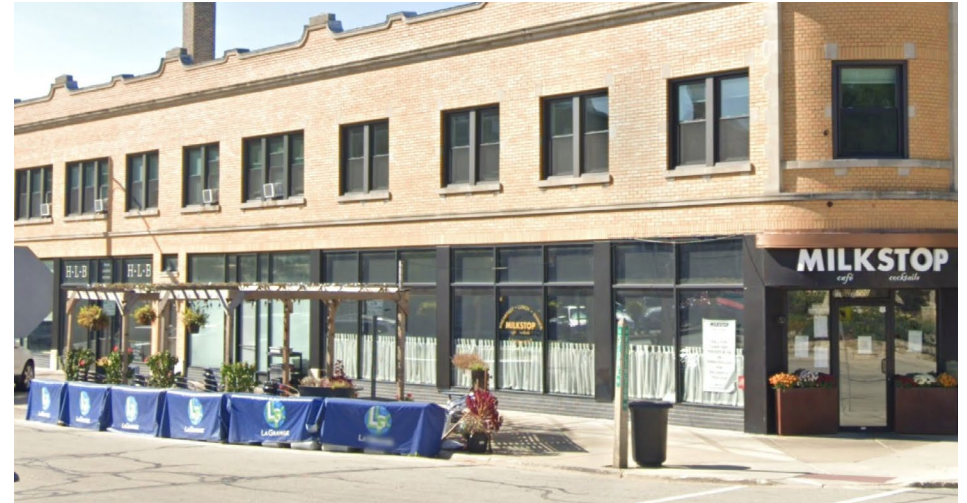
Opportunity location within the West End for a parklet (Burlington Avenue and Stone Avenue) Image Sources: Google Streetview, 2022
