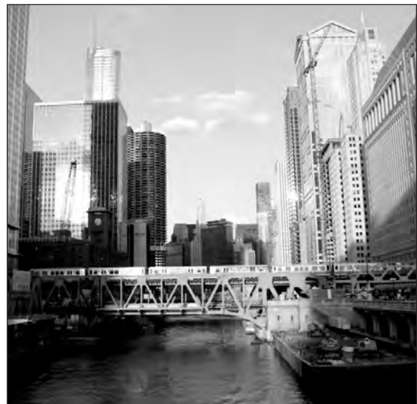
By coordinating critical CTA track work at the Tower 18 junction with CDOT's reconstruction of the 90-year old Wells Street Bridge, both agencies achieved cost savings and reduced the work's impact on the roughly 40,000 CTA rail customers who travel across the bridge each weekday.
