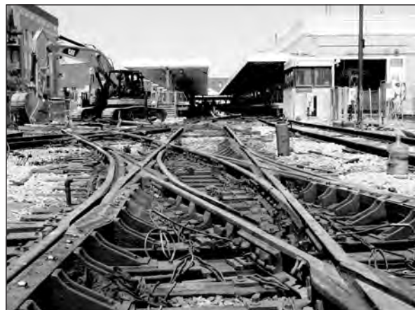
This summer, the Kimball Brown Line terminal was closed for nine days to replace track and rail system components that were 50 years old and beyond their useful life.
