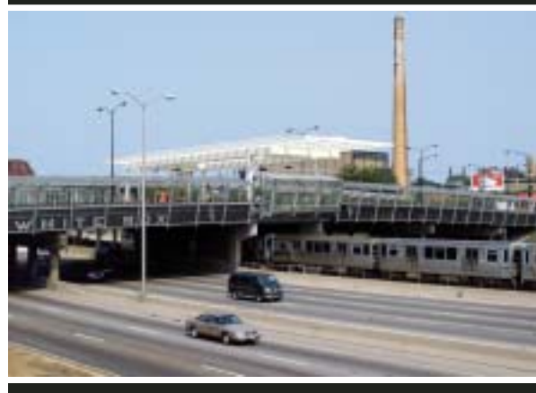
The newly renovated Sox-35th station on the Red Line.
