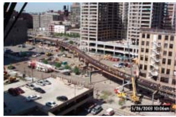
The curved track at Harrison Curve was removed and replaced with a new, more linear track. These before and after photos show what the CTA can accomplish in a weekend.
