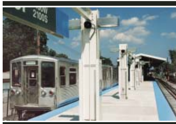
A train arrives at the newly renovated platform at Kostner station, part of the Cermak (Douglas) rehabilitation project.
