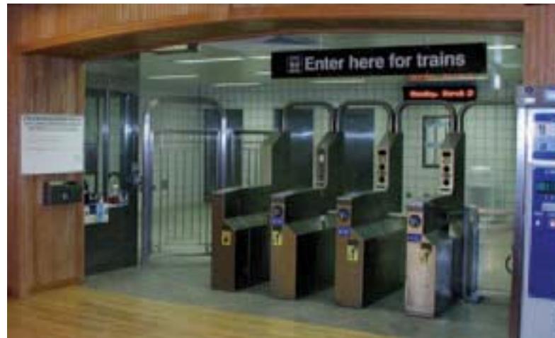
As seen in the fare area, parts of the original station were incorporated into the newly renovated Kedzie station on the 54th/Cermak branch of the Blue Line.
