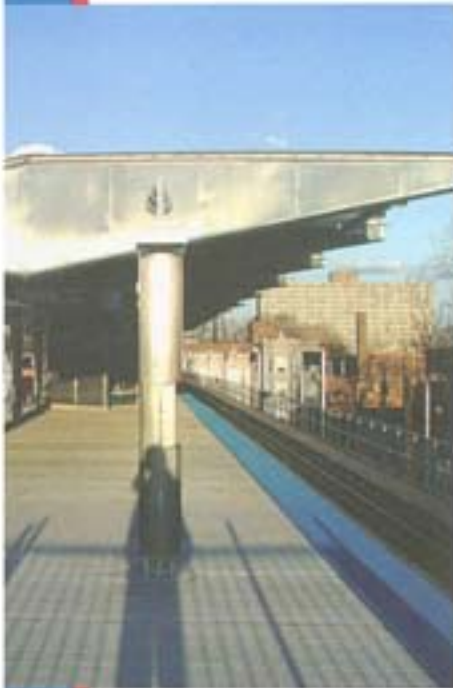
The renovated platform at the Kedzie station on the 54th/Cermak branch of the Blue Line features a stainless steel canopy.
