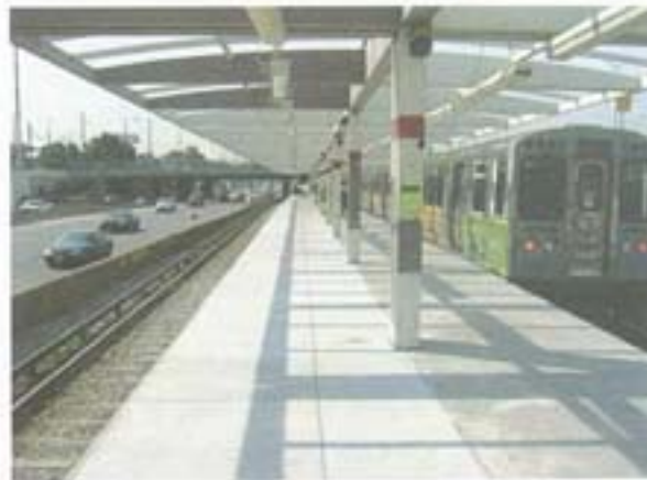
A new concrete platform is one of the upgrades at the Garfield station on the Red Line as part of the rehabilitation of the Dan Ryan branch.
