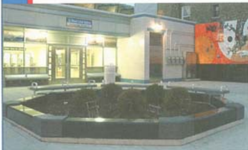
Improved lighting at the Blue Line's newly renovated Damen station on the 54th/Cermak branch lights up the neighborhood at dusk.
