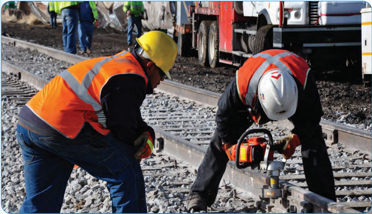
Metra signal maintainers apply a bond wire to a join in the rail.
