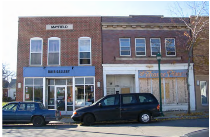
Many of the buildings along Sheridan Road are currently being renovated. This photo shows two building facades during an early stage of renovation.
