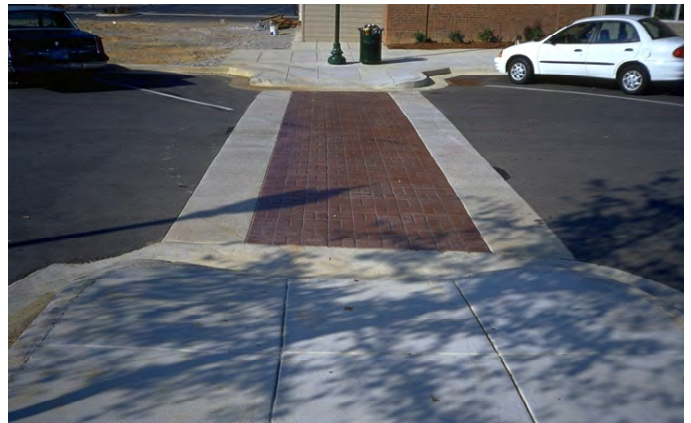
Bulb-outs shorten the crossing distance and provide safe areas for pedestrians to stand.
