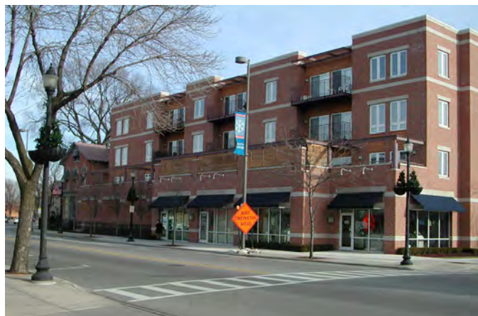
This mixed use building incorporates quality materials, such as brick, concrete, and wood. It also has a flat roof with a parapet, which is preferred over other roof types.
