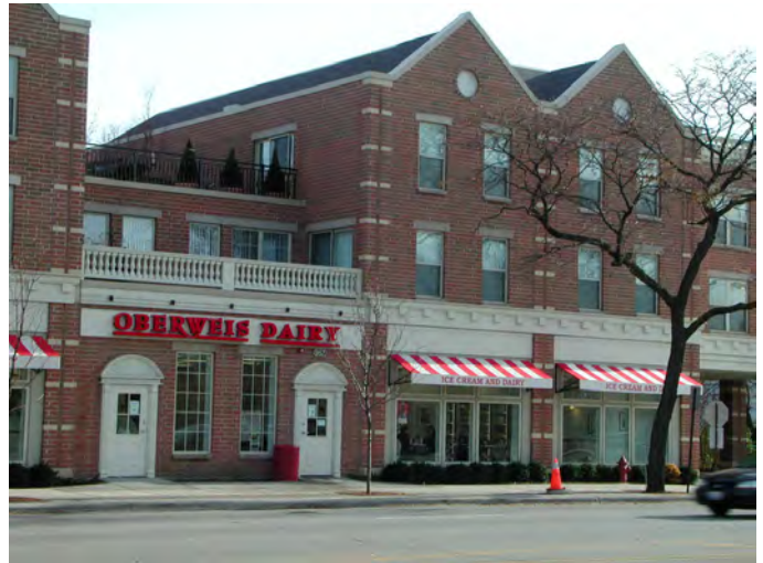
This building has an occupied first floor street facade and an expression line above the ground floor.
