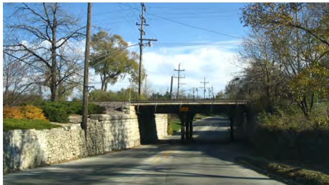
Foss Park Avenue runs beneath the Metra/UP-North Line.
