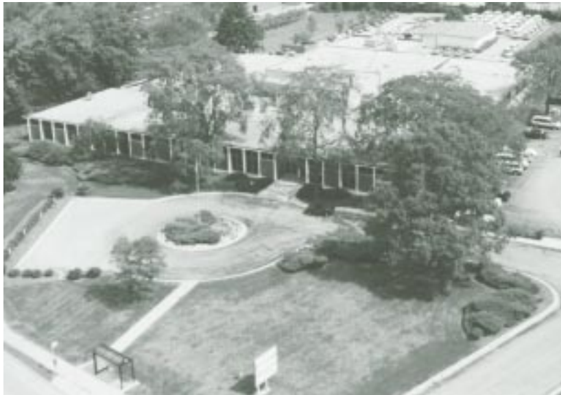
Pace Headquarters Facility in Arlington Heights.
