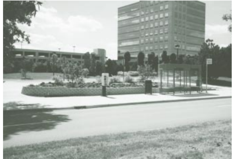
Elk Grove Park-n-Ride lot was completed in September, 1998.
