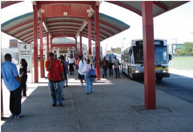
The Pace Transportation Center in Harvey is one of the heaviest used facilities in our system.
