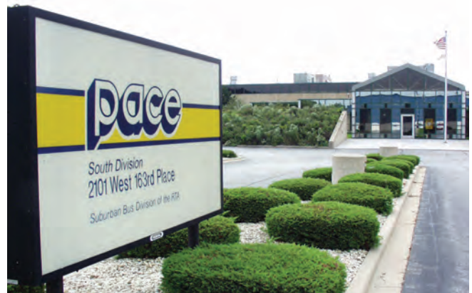
Pace South Division in Markham is one of our largest facilities, with 191,000 square feet.
