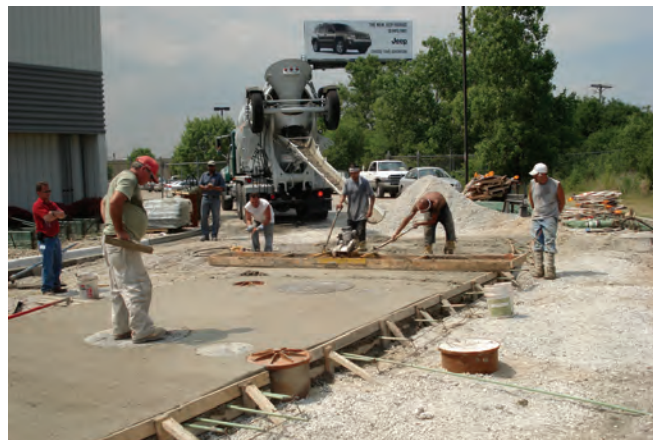
Pace completed concrete replacement at its Southwest Division in Bridgeview in 2007.
