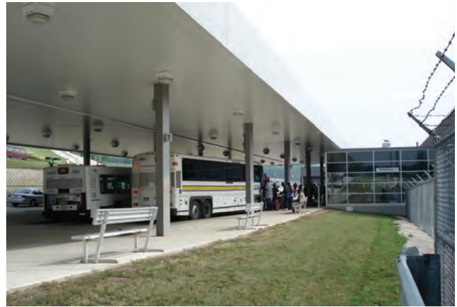
Pace constructed two transportation centers at the UPS facility in Hodgkins in 2003. This facility continues to carry over 2,000 employees to the location each day.
