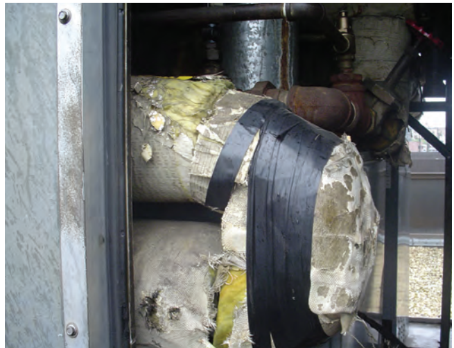
Pace replaced 7 out of 8 boilers at its Heritage Division. These boilers were beyond their useful life.
