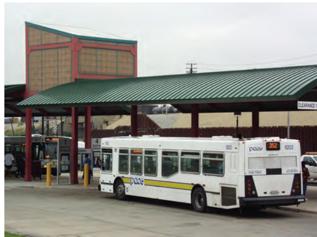
Pace constructed the Harvey Transportation Center in 1999. It is the most heavily used facility in our system.
