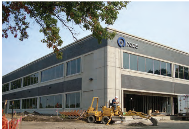
Construction is nearing completion of Pace's new administrative office building.
