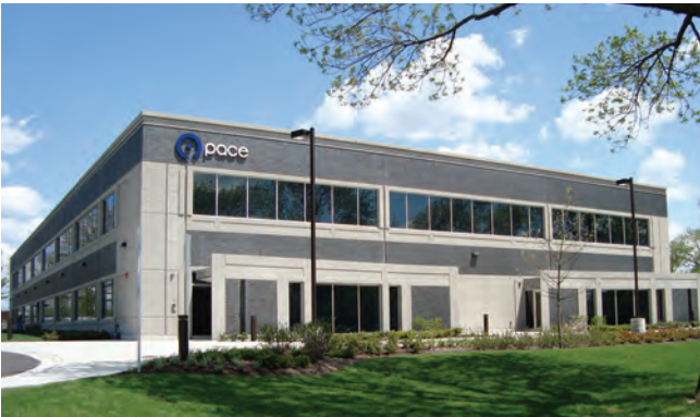
Pace completed the construction of its new administrative headquarters building and moved in on April 27, 2009.
