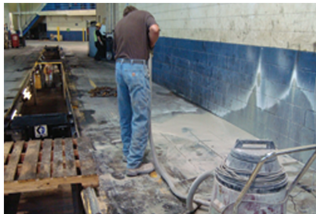
Due to aging equipment, Pace replaced a broken grease line at South Division in 2011.
