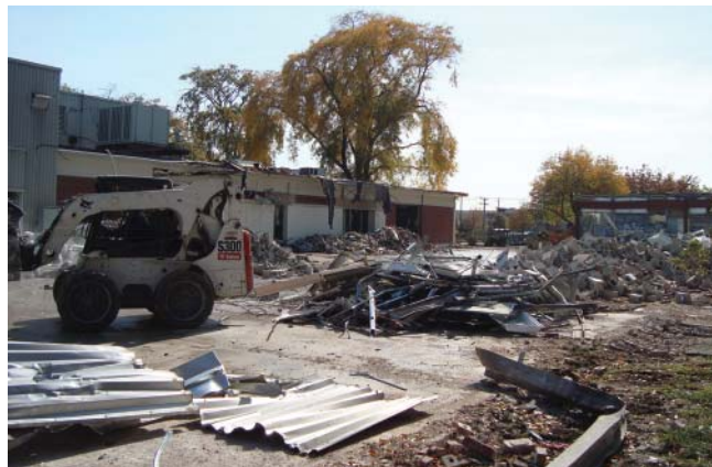
Pace demolished its old Headquarters building in 2010.
