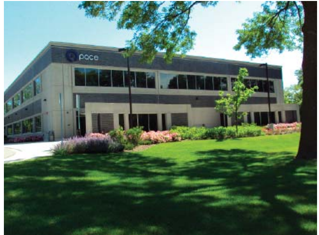
Pace opened its new Administrative Headquarters building in spring of 2009.
