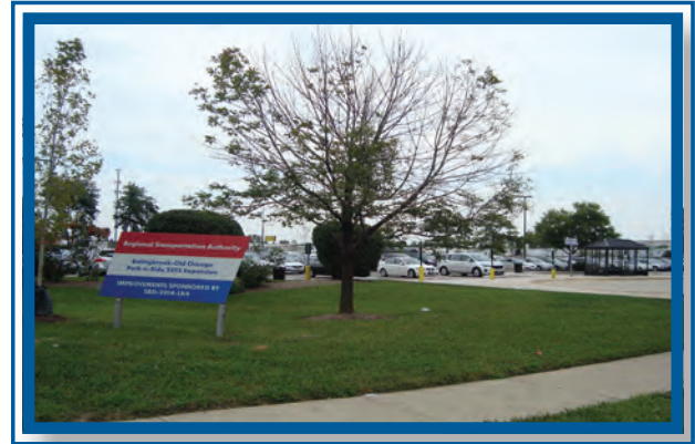
Pace is completing the expansion of Bolingbrook Park-n-Ride at I-55 and Route 53 to accommodate increases in ridership from the Bus on Shoulder service. This expansion will add 71 additional spaces for a total of 219 spaces.
