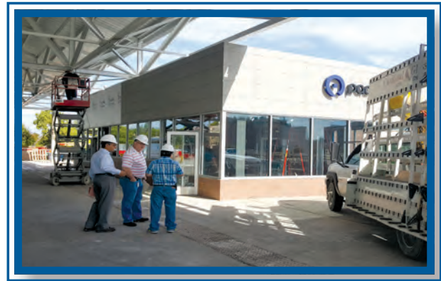
In 2016, Pace will complete a major mid-life renovation to the Pace Transportation Center in Elgin including the construction of a new passenger building.
