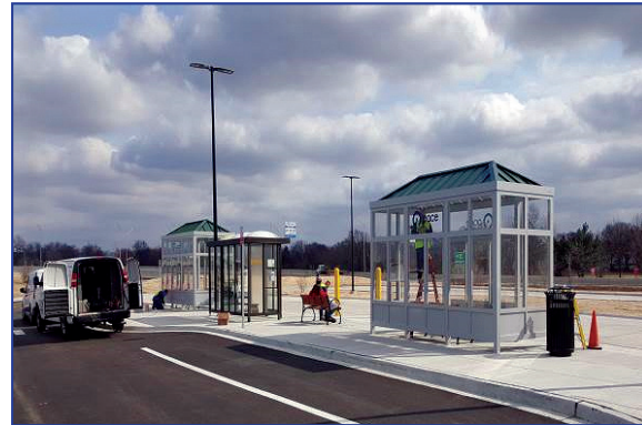
Heated bus shelters were installed at the new I-25 Park-n-Ride, which supports the Bus On Shoulder service on I-90.
