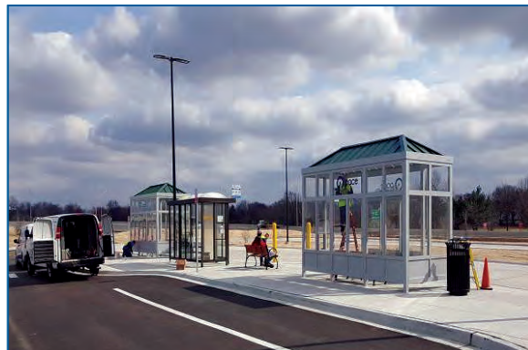
Heated bus shelters were installed at the new I-25 Park-n-Ride, which supports the flex lane operation on I-90.
