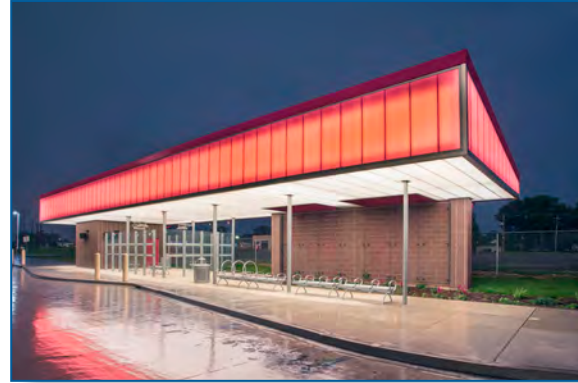
Work on the Bridgeview Transit Center was completed in 2019.
