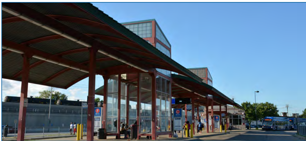
Pace's Harvey Transportation Center, located adjacent to the Harvey Metra Station, provides a key transfer point for Pace bus routes that serve the entire south suburban region.
