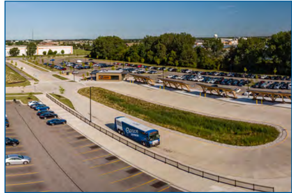
The parking lot at the new Plainfield Park-n-Ride is now operational, providing additional parking for the I-55 Bus on Shoulder service.
